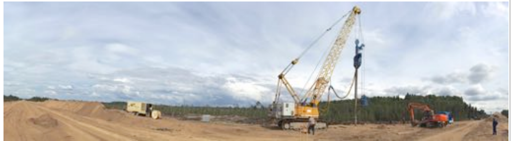
BC1 rig with B27 vibroprobe installing 80 cm to 160 cm diameter sand columns.
