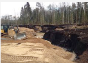
Dozer applying the sand fill
