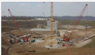
Two rigs working on slope
