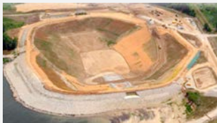
Aerial photo of excavation
