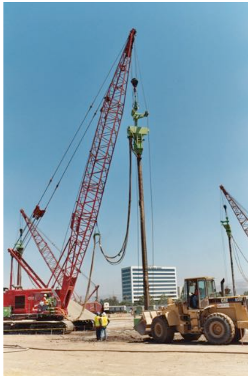
View of two V23 Dry Bottom Feed rigs. In background: Irvine Medical Center
