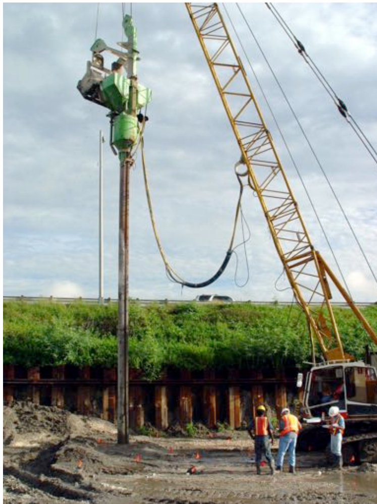
Skip Bucket Rig on Liebherr 843 crane
