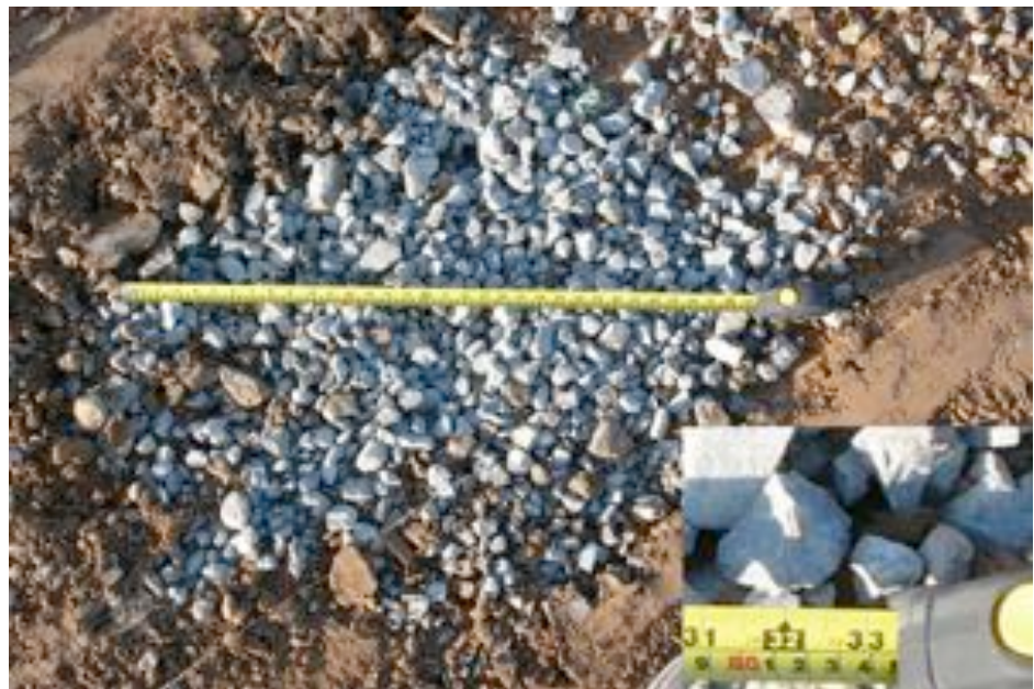
Dug out Stone Column, measuring approximately the required 85 cm.
