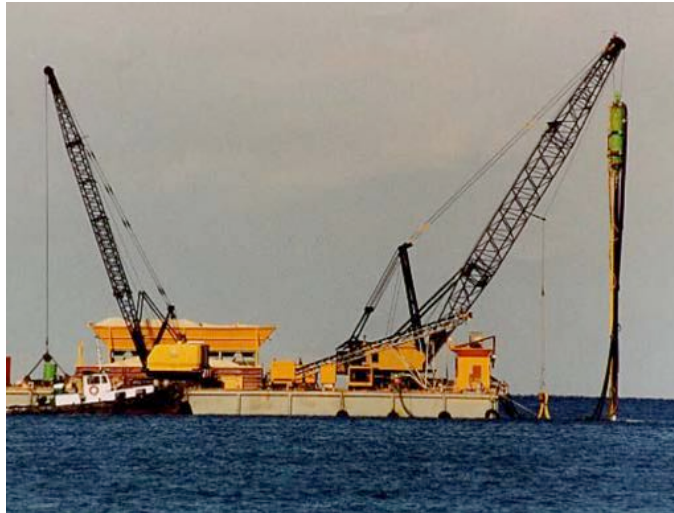
Barge with Double Lock Gravel Pump Vibro Rig (right)
