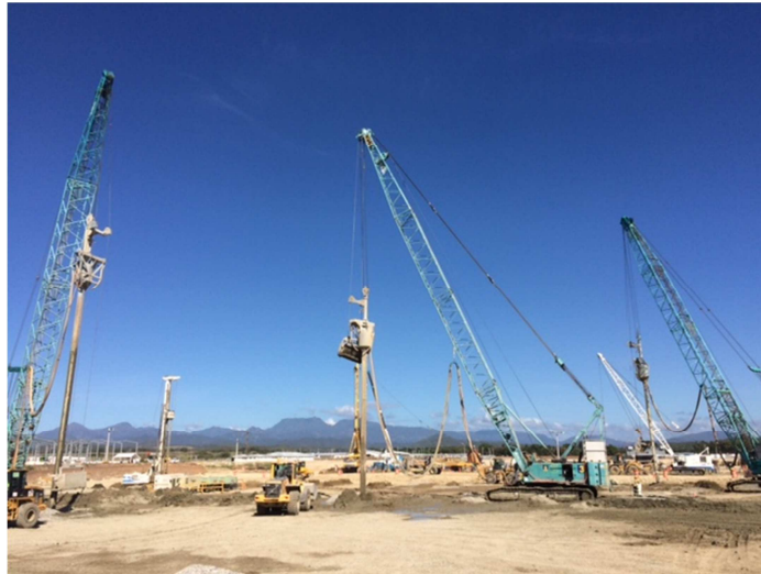
3 Vibro B27 Dry Bottom Feed rigs working on site
