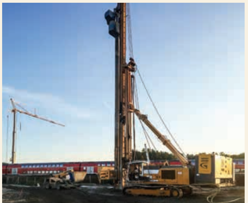
Flyover Heldenstein, Highway A94, Germany (2016): Dry Bottom Feed Stone Columns installed with BL1 attached to Liebherr drill rig carrier
