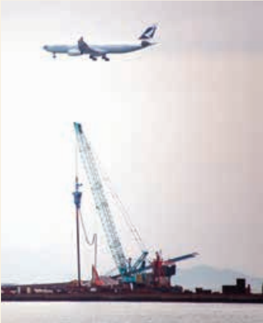
Marine Stone Column works under very strict Airport height restrictions.
