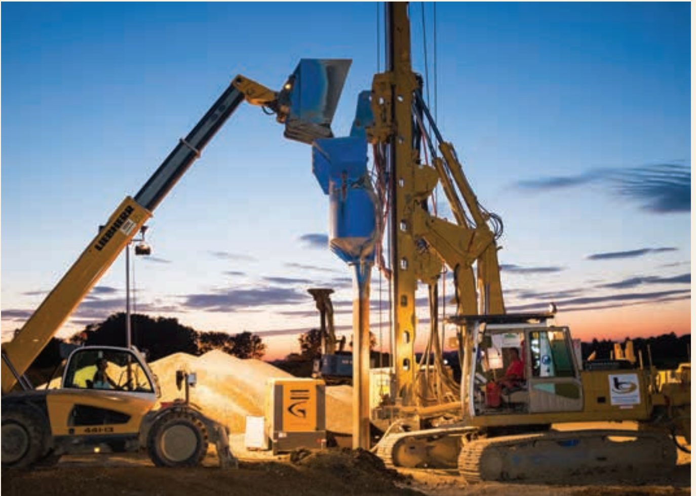
Foundations for railroad-road flyover Mue30, Schwindegg, Germany (2015): BL3 Bottom Feed Stone Columns rig, attached to BAUER BF12
