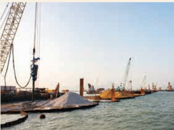
Bottom Feed Stone Columns inside 31 m diameter caissons. 57 columns are installed in each caisson.
