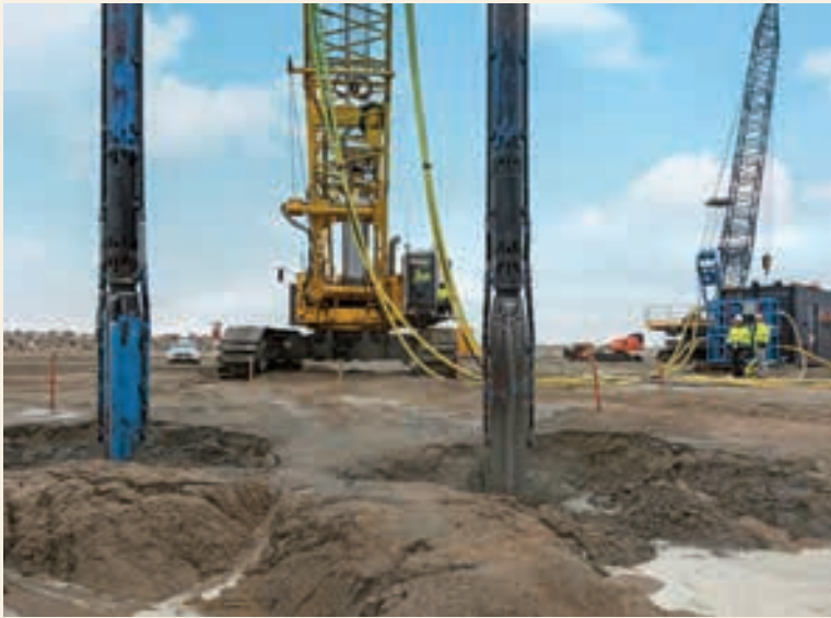
Port of Calais, France: Vibro Compaction in Tandem arrangement.
