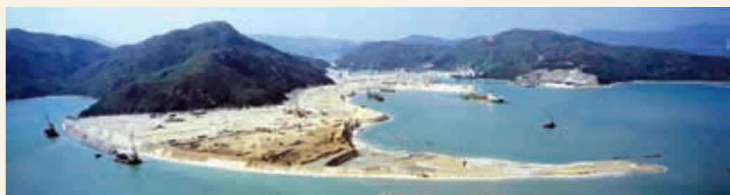
The world's largest Vibro Compaction project before Dubai's Palm islands: 40 million m 3 marine sand, with compaction depths up to 40m. Hong Kong Penny's Bay project (Disney Hong Kong) 2001-2003
