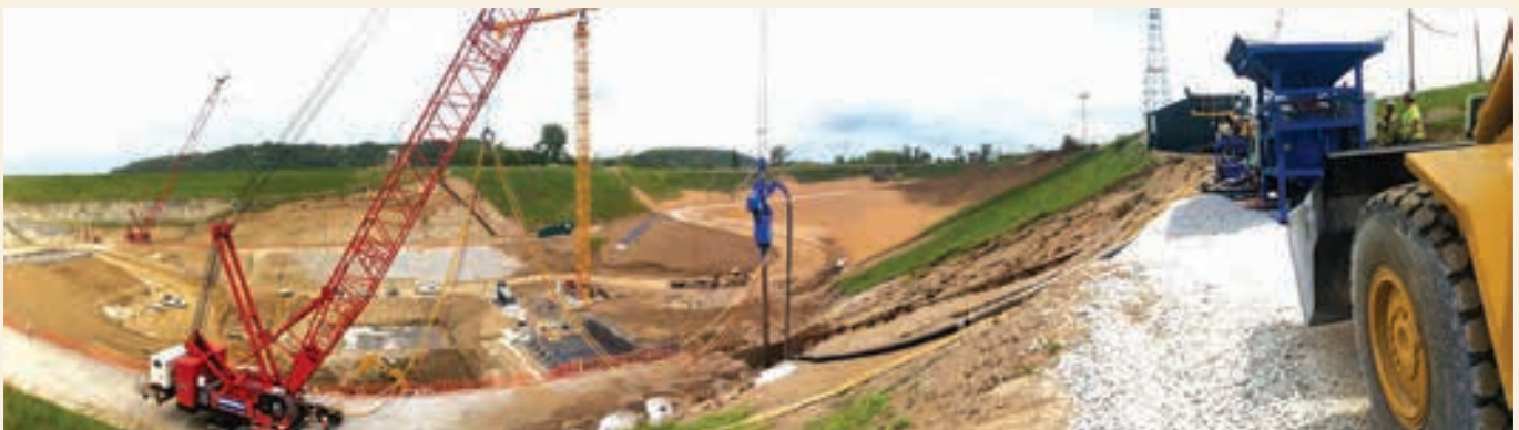
Cannellton Lock, USA (2011): Dry Bottom Feed Stone Columns installed with GP1 pneumatic stone transport rig
