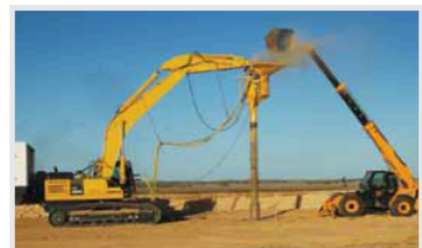
The vibroflot is frequently moved up and down in order to form and compact a column. Thereby, the surrounding ground is horizontally compressed and improved. The column is able to support high vertical loads.
