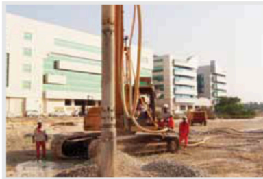
The vibroflot penetrates and 'washes' the hole in preparation for the stone transport within the hole.
