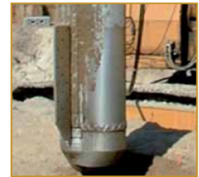
The vibroflot is frequently moved up and down in order to form and compact a column. Thereby, the surrounding ground is horizontally compressed and improved. The column is able to support high vertical loads.
