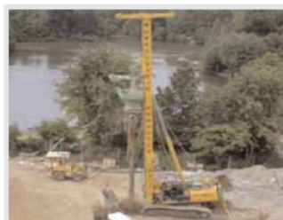
The stones are introduced via a tremie pipe along the vibroflot and the aid of pressurized air.
