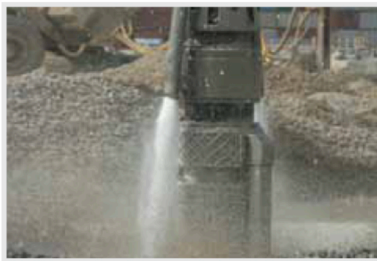
During introduction of the stones, water and air are flushing in order to create a positive flow for the stone transport.
