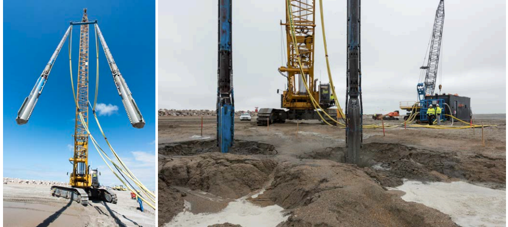
Tandem Rigs with B41 vibroflots working in the compaction trial area
