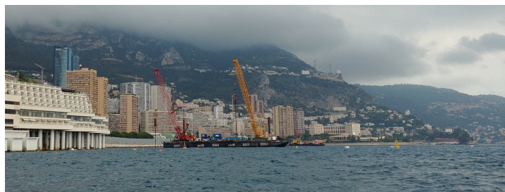
Top: Two cranes with B41 vibroflots working from one barge. Right: The rubble fill material that needed compaction.
