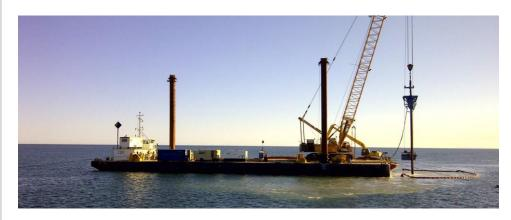
The Boleo Marine Terminal, located at Santa Rosalia, Baja California Sur. The facilities consisted of a 350m wharf and four mooring dolphins. The wharf and dolphins were supported on driven open-ended pipe piles found-ed a specified length into sedimentary bedrock. The granular soil above the bedrock was susceptible to liquefaction and ground treatment was specified. As this portion of the project was design build.
