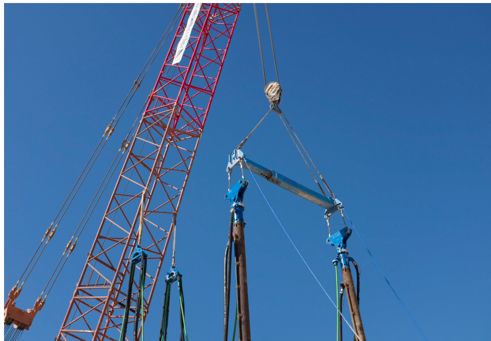
Typical Tandem setup on crawler crane
