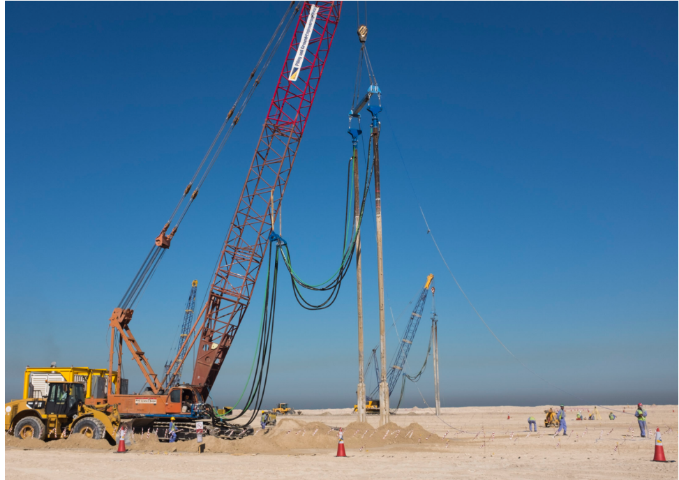
Two TC1 Tandem Rigs with B41 vibroflots
