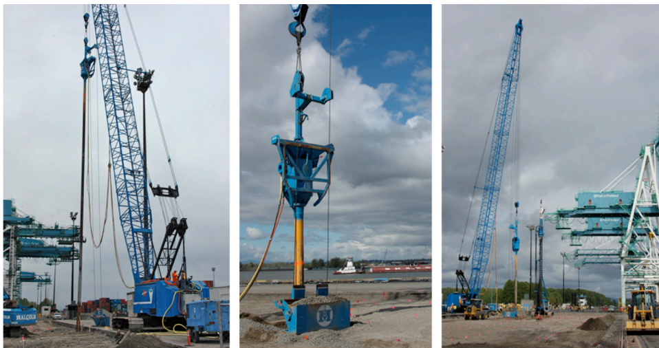
Vibro B27 Dry Bottom Feed rig, left: ready for 100 ft penetration depth, middle: at target depth
