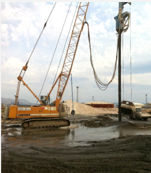
22 m capacity BC1 Bottom Feed Stone Column rig.
